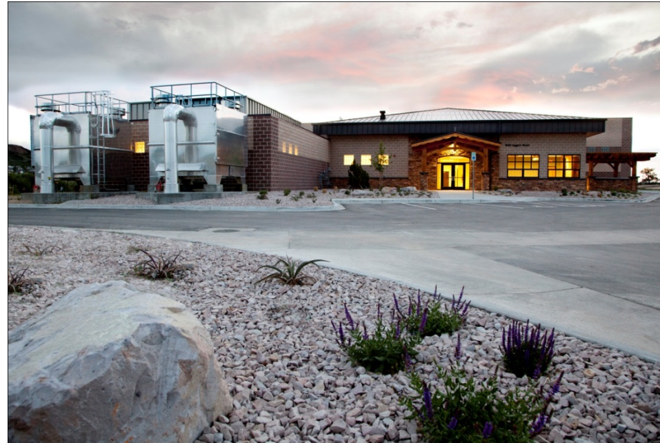
Setting a good example Our new Plum Creek Water Purification Facility
