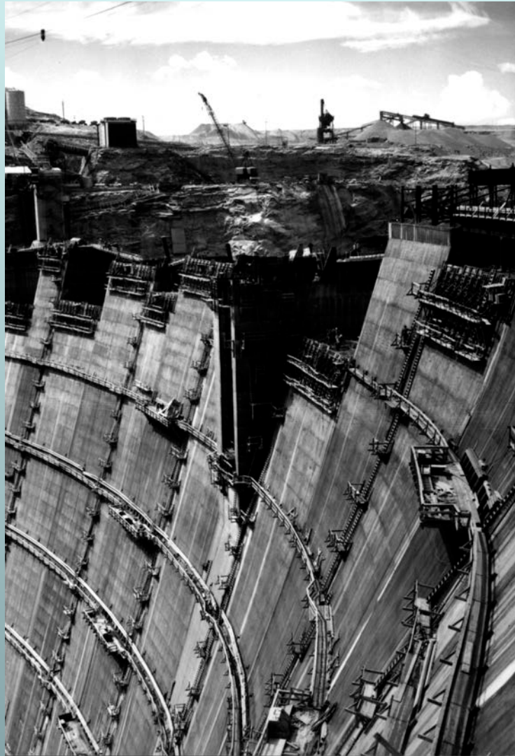
Glen Canyon Dam Under Construction
