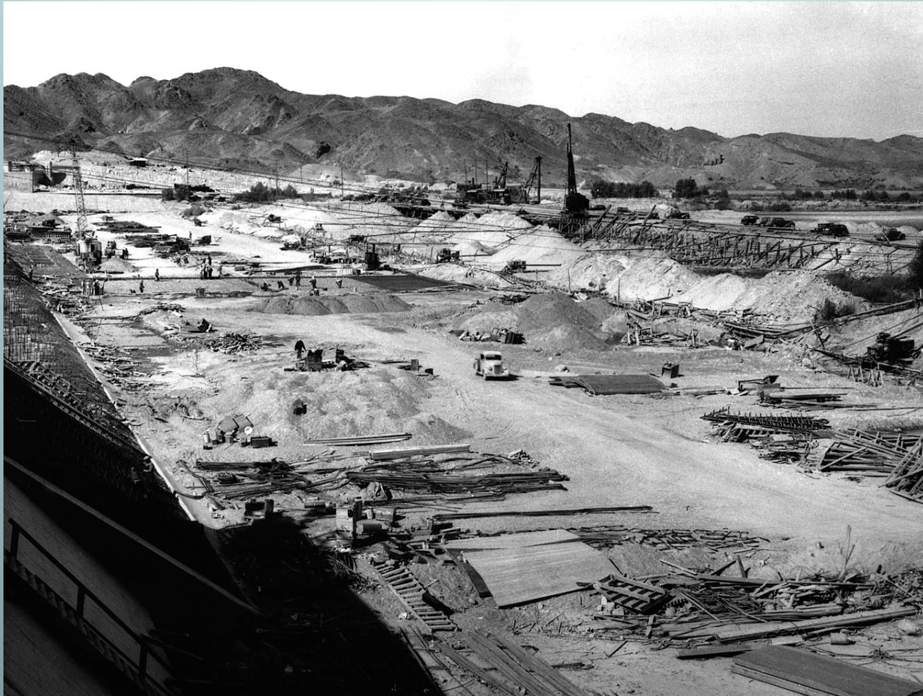
All American Canal Under Construction
