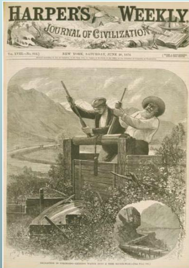
Harper's Weekly was one of the most popular illustrated newspapers of the 1800s. In this 1874 edition, the Union Colony and Colorado irrigation made the front page in an engraving captioned "letting water into a side sluiceway" in reference to what are now called "headgates."
